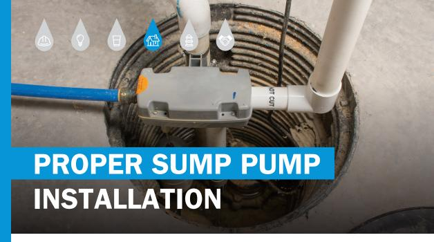
Homeowners should be aware that connecting sump pumps to the sanitary sewer is unauthorized, plus it can cause big problems!
